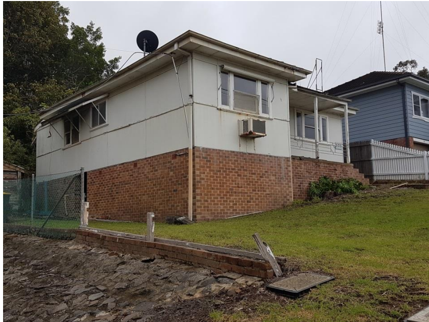
Figure 2 – Existing dilapidated cottage
